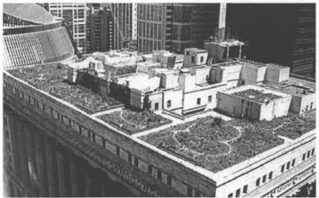
FIGURE 5-18 City Hall in the center of Chicago's downtown was retrofitted with a green roof to reduce the heat island effect, remove airborne pollutants, and attenuate stormwater flows as a demonstration of innovative stormwater management in an ultra-urban setting. SOURCE: Conservation Design Forum.
